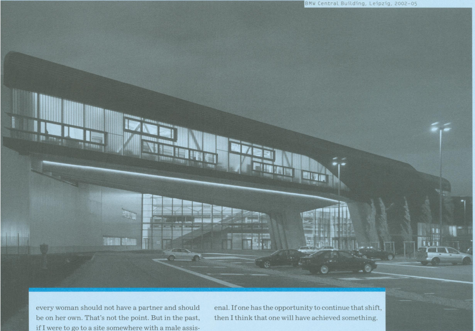
BMW Central Building, Leipzig, 2002–05
